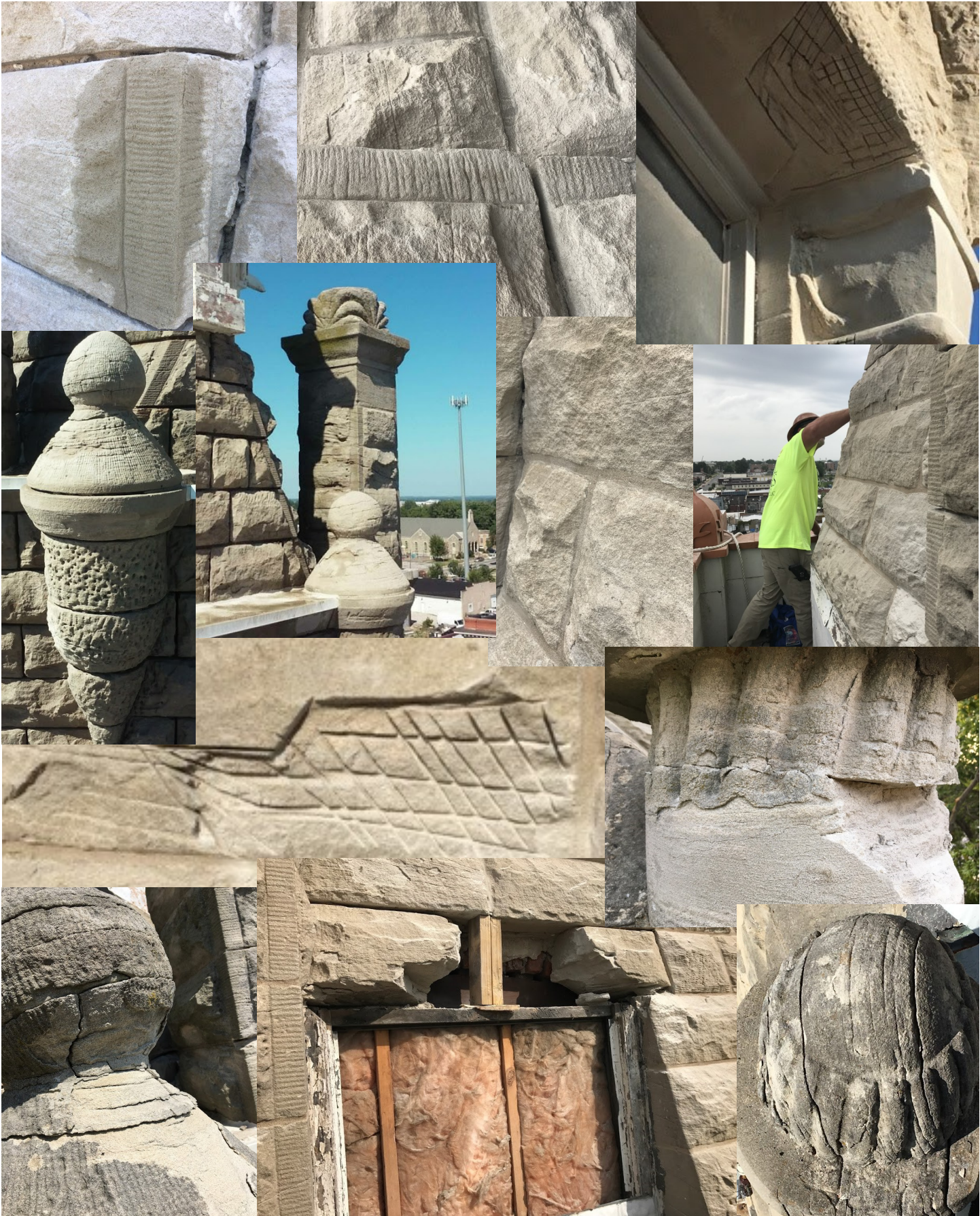
Stone: Cleaning, patching, tuck-pointing and 100% stone consolidation treatment.
